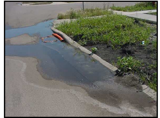
Inlet protection installed correctly
